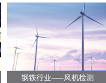
钢铁行业——风机检测
