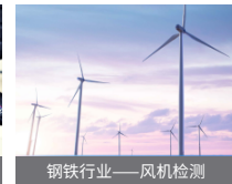
钢铁行业——风机检测
